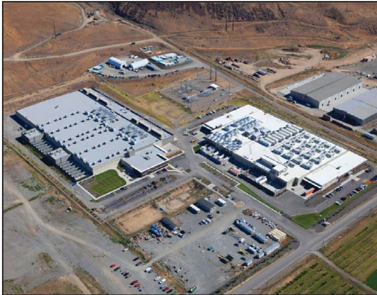
The Intergate.Columbia data center campus in Wenatchee, WA.
